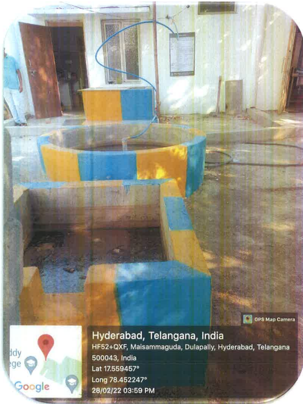
Biogas facility to deal with Kitchen waste
