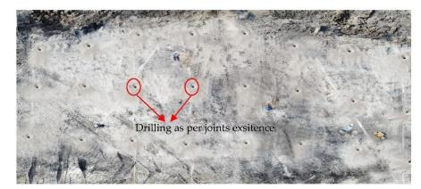
Figure 11. Bench photograph after drilling.
